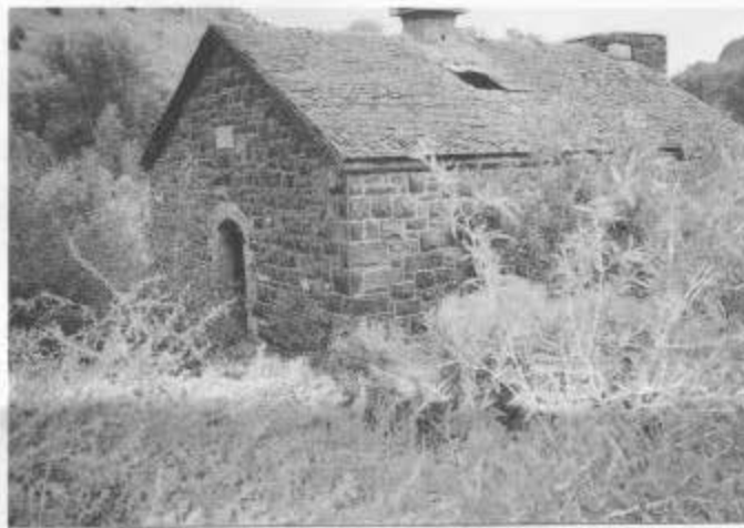
Lava Pump House, June 27, 2001. (Photo by Robert Hayes.)
