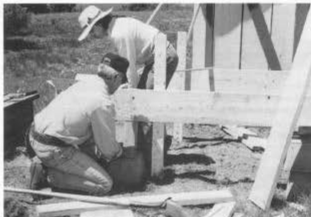
Bob Akers and Noreen Breeding level the frame of the new back porch on the Cumbres section house (session A).
