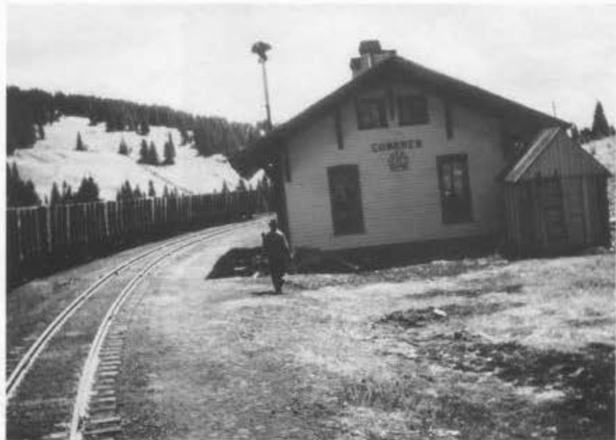
View from the parlor car of the westbound San Juan after the train has pulled out of the Cumbres station on May 16, 1950, and showing the west elevation of the station. Note the string of high-side gondolas. (Photo by Donald G. Hills, collection of Wayne D. Hills.)
