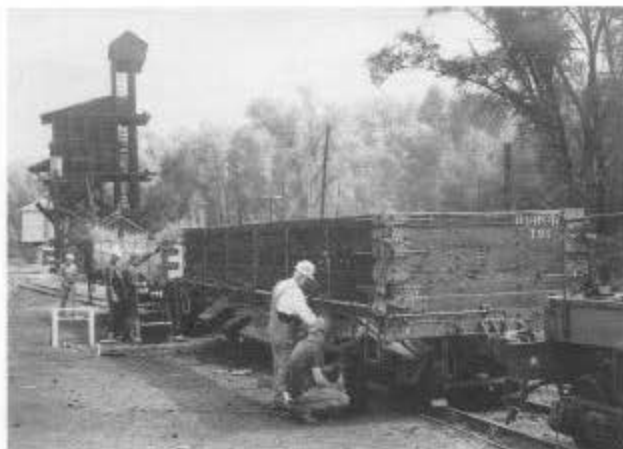
Drop bottom gondola 791 in the Chama yard before the volunteers begin disassembling it in session D. The car will be a 2002 restoration project. (Photo by Tom Cardin.)
