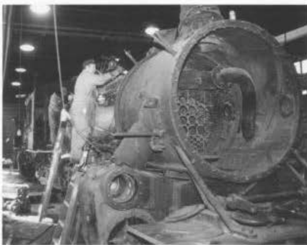
Jose Torres (l) and Ricky Rivas apply red primer to the boiler of 484. New valve cages can be seen installed. The smokebox flue sheet has been checked and is ready for flues (January 2002).
