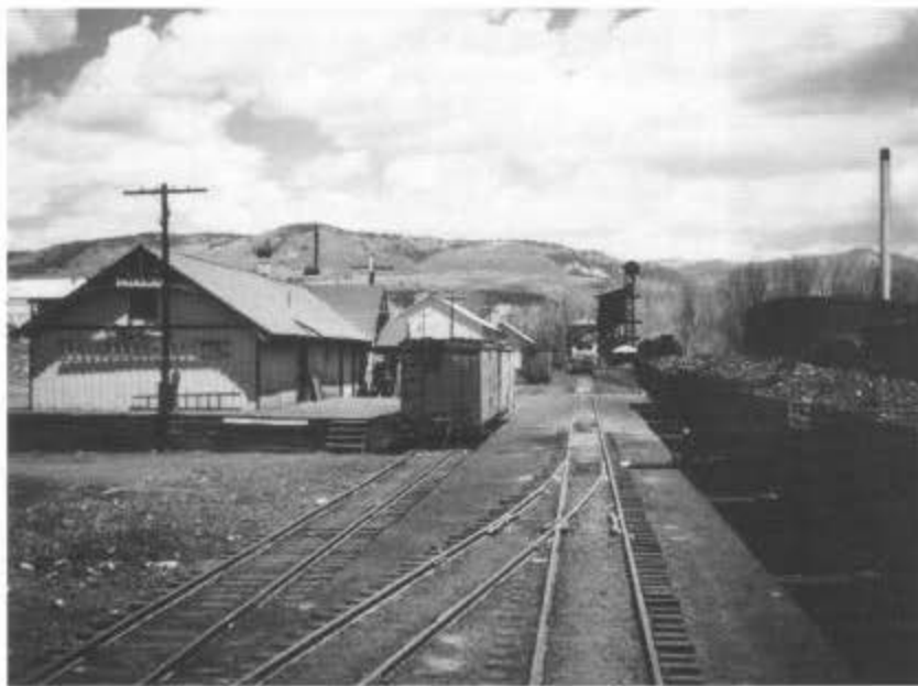
Looking north in the Chama rail yard from the departing San Juan on May 16, 1950. Note the fire ladder hung on the wall of the depot. Two D&RGW short refrigerator cars are parked at the depot's loading dock. (Photo by Emery B. Smith, collection of Wayne D. Hills.)
