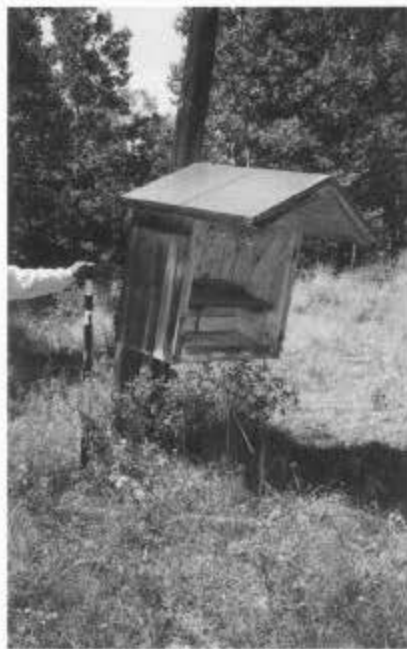
Pole-mounted phone box at Toltec Siding.
