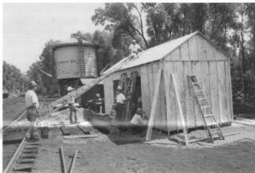
In session D team members work on the new roof and nail the battens to the sides of the new speeder shed located south of the Chama water tank. The shed will house historic Fairmont speeders 04 and 013, which are being restored.
