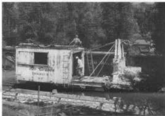
Below the Chama engine house, volunteers work on derrick OP's roof, operator's house, and boom A-frame support structure to stabilize the derrick until a complete "from the wheels up" restoration is done (session E). (Photo by George Swain.)
