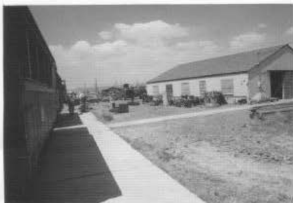
Overall view of Fort Knox and the concrete pads along the repair in place (RIP) track at Antonito (session C).
