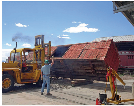
Step 5: Not all the salvage parts are easily accessible. A forklift helps get the crew to the underside.
