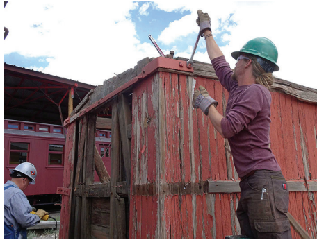
Step 2: Salvage the metal parts that might be useful on Boxcar 2332.
