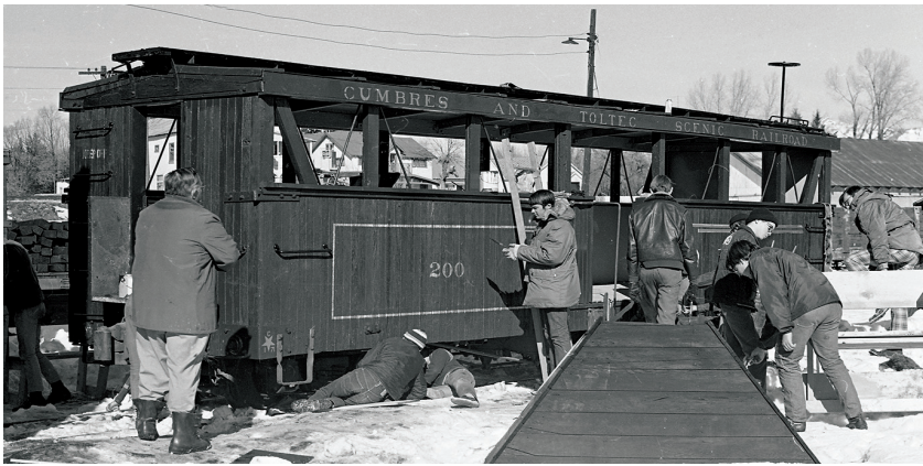
Volunteers in Chama work on a cold day in January 1971 converting D&RGW Boxcar No. 3339 to C&TS Box Car Coach No. 200.
